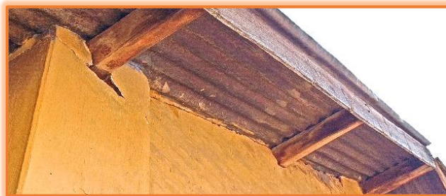
Figure 60 Cracks at beam column joint library, nardipur
