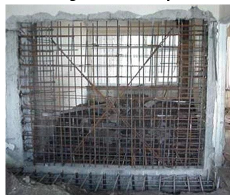
Figure 177 New Shear Walls
