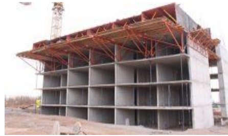
Figure 182 Tunnel Formwork System
