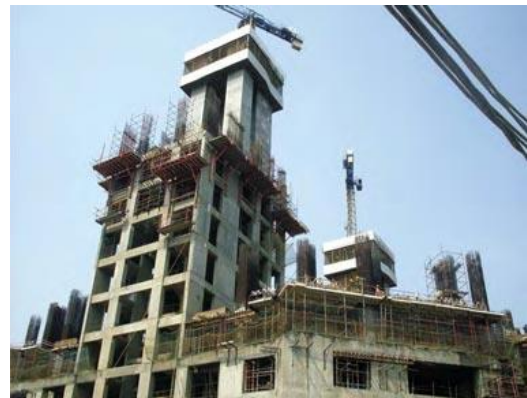
Figure 188 Palais Royale–The Tallest Building in India under construction with M-80 Concrete Columns in Self-compacting Concrete
