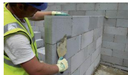
Figure 186 Thin Joint Masonry Technique
