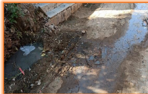
Figure 46 Inadequate drainage system
